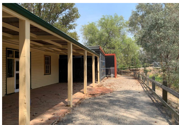
Figure 2B – Existing building (rear)
