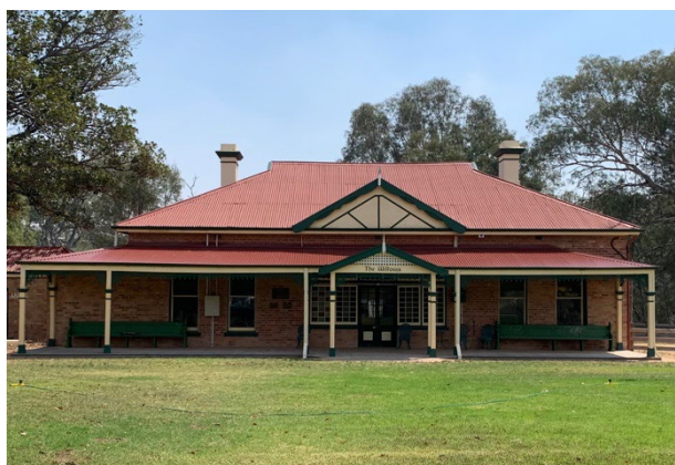
Figure 2A – Existing building (street) 4
