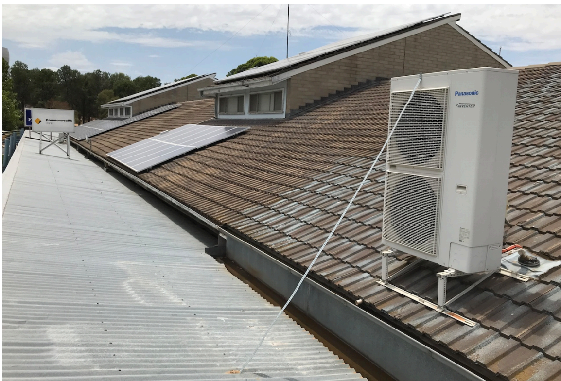
Typical view of existing verandah roof to Brolga Place shops looking northeast (Council building similar). Box gutter depth varies from flashing line behind main building fascia gutter (forefront) to full depth to main building wall (beyond). Some advertising structures are located on the verandah roof that will have to be temporarily removed and relocated upon completion of the new verandah.
