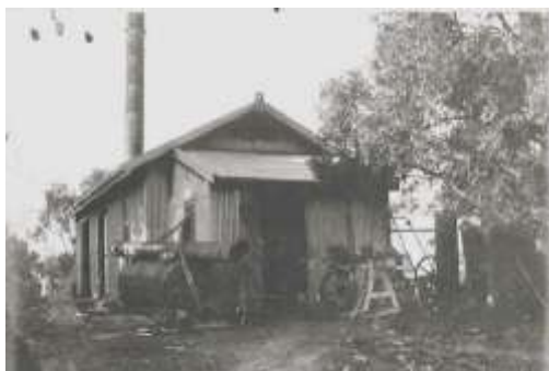
The old pump station demolished in 1964
