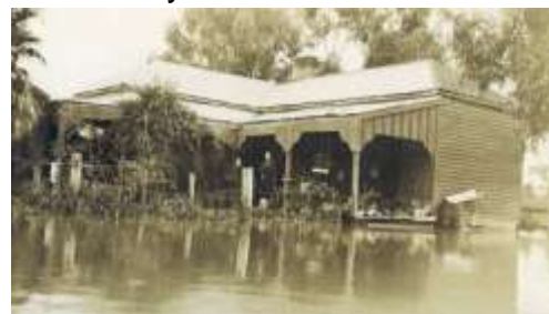
Chapman residence surrounded by floods in 1931
