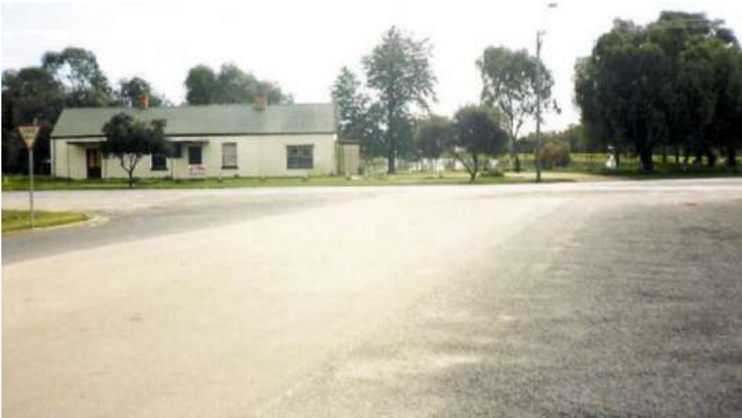
Chapman's, or Creedy's flats before demolition, once the residence of James Mahood, and residence and surgery of Dr Robinson.
