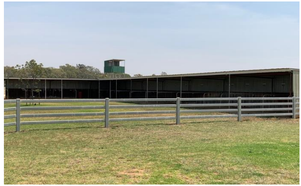
Figure 7 – Marshalling area and stables
