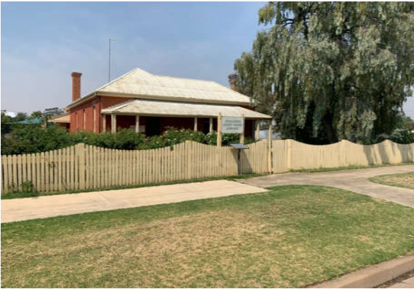
Figure 3A – Existing building 4
