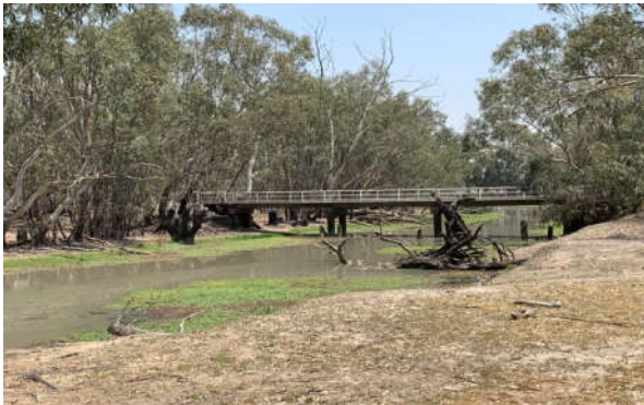
Figure 10 – Bridge looking west
