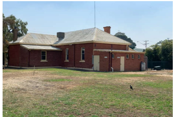
Figure 3D – Rear of existing building
