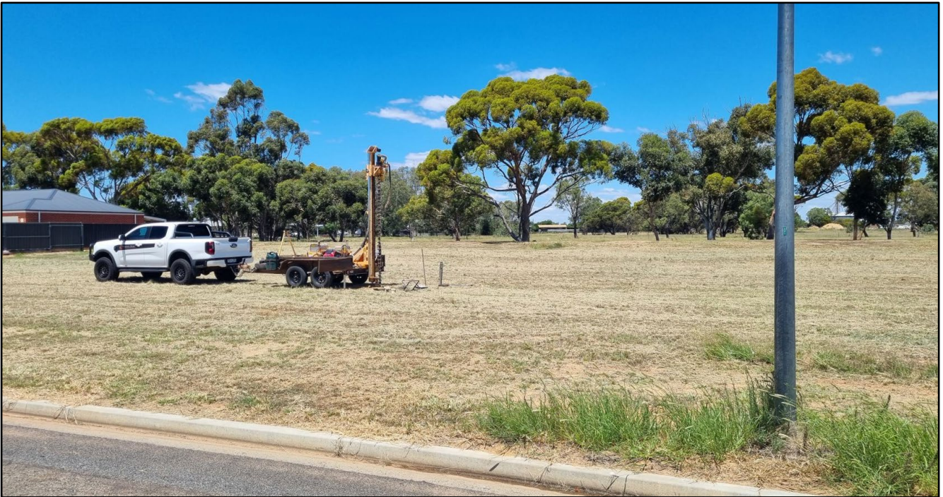
Site Photo – BH1 Looking South (18/01/2024)
