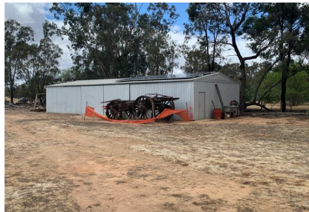
Figure 3H – Other buildings
