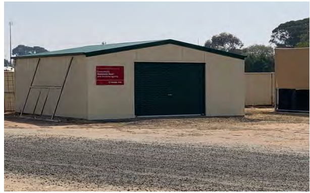
Figure 13 – Machinery storage shed
