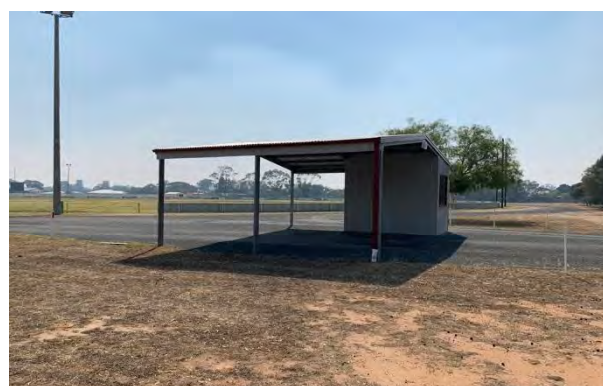
Figure 7 – Canteen (part of main building)
