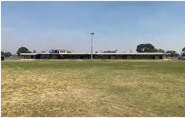
Figure 18 – Main building from oval
