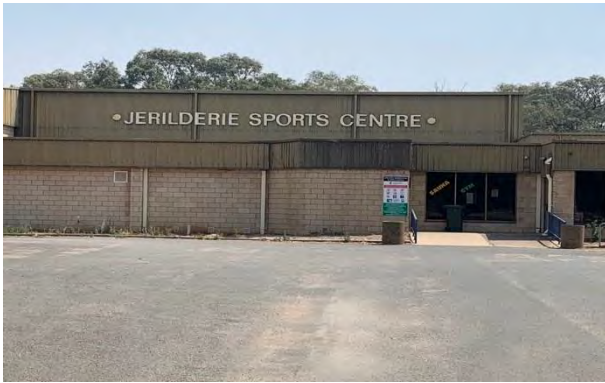
Figure 2 – Main building and carpark 4
