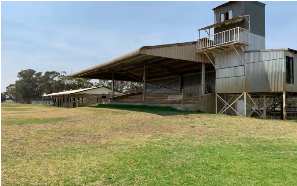
Figure 2 – Grandstand and control tower 5
