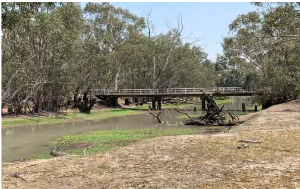
Figure 10 – Bridge looking west
