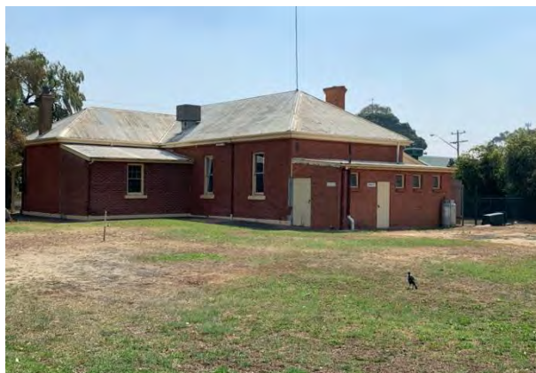
Figure 3D – Rear of existing building
