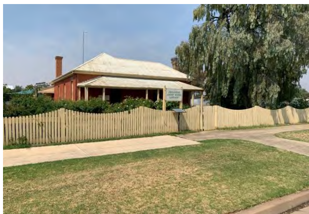
Figure 3A – Existing building 4
