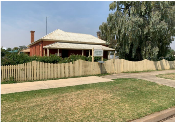
Figure 3A – Existing building 4
