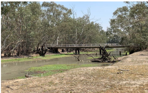
Figure 10 – Bridge looking west
