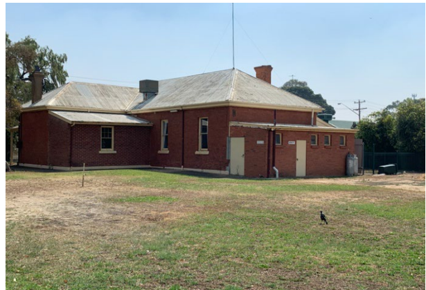
Figure 3D – Rear of existing building
