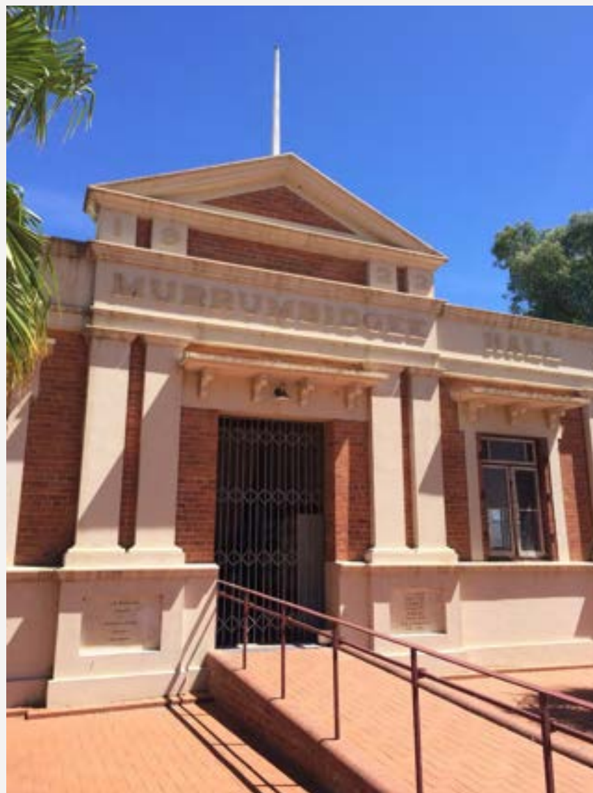
Former Murrumbidgee Shire Hall
