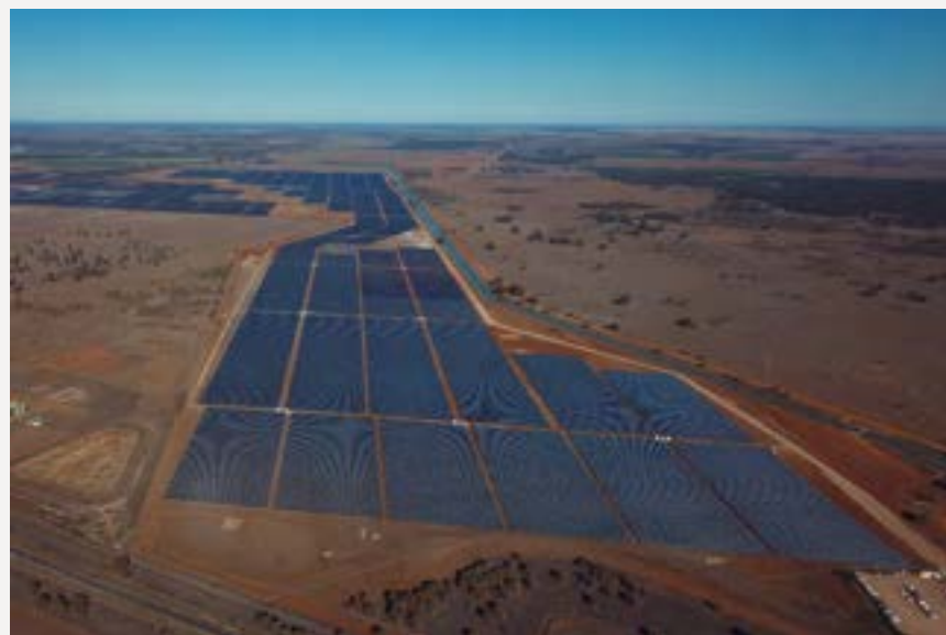
Coleambally Solar Farm
