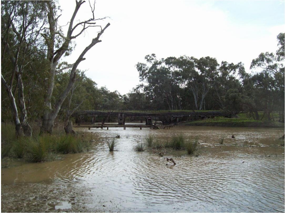
Photograph 1 Looking downstream towards the Billabong Creek rail bridge (R1)
