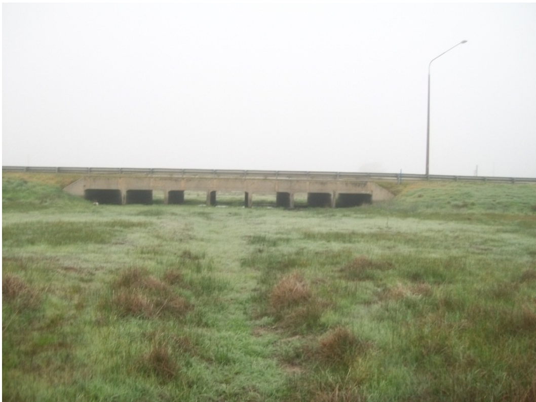
Photograph 4 Wangamong Creek Newell Highway culvert (C2)
