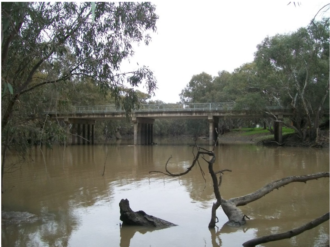
Photograph 2 Looking upstream toward the Billabong Creek Newell Highway Bridge (B1)
