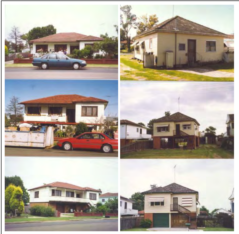
Plate 29 Examples of houses before (top image), during (middle image) and after (bottom image) house raising (photos courtesy of Fairfield City Council)
