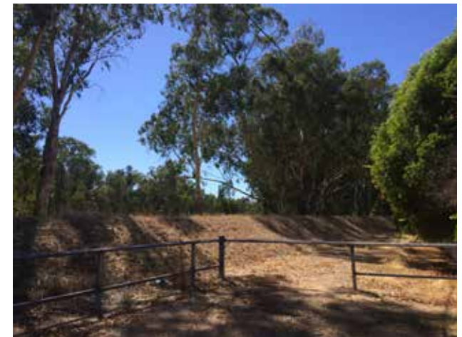
Figure 10 - Existing Flood Levee Bank
