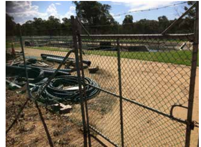
Figure 9 - Wastewater Treatment Facility
