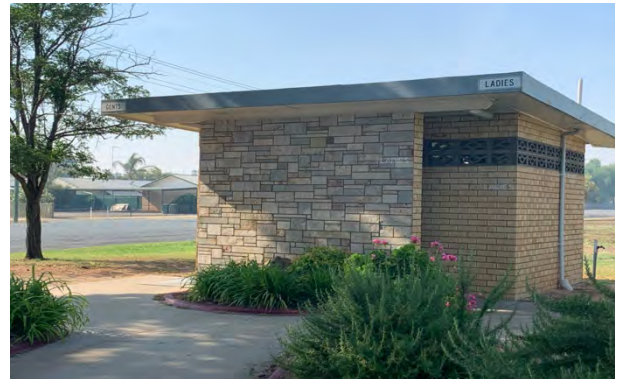
Figure 8H - Existing amenities' building
