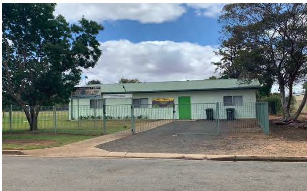
Figure 4 – Existing community facility 4
