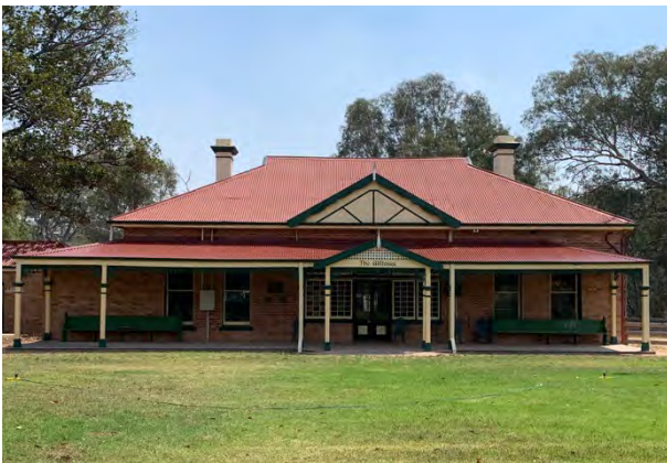
Figure 2A – Existing building (street) 4
