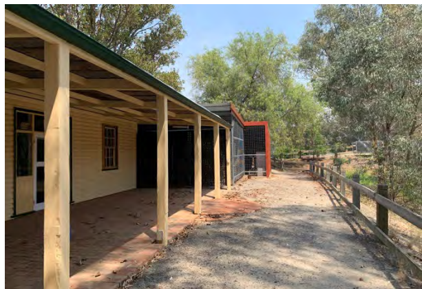
Figure 2B – Existing building (rear)
