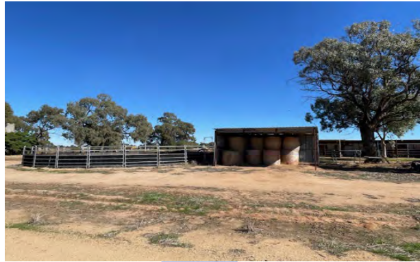
Figure 15 – Corral and shed at Darlington Pt
