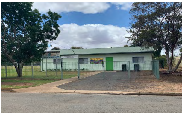
Figure 4 – Existing community facility 4
