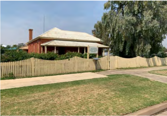
Figure 3A – Existing building 4
