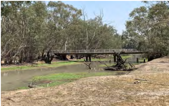
Figure 10 – Bridge looking west
