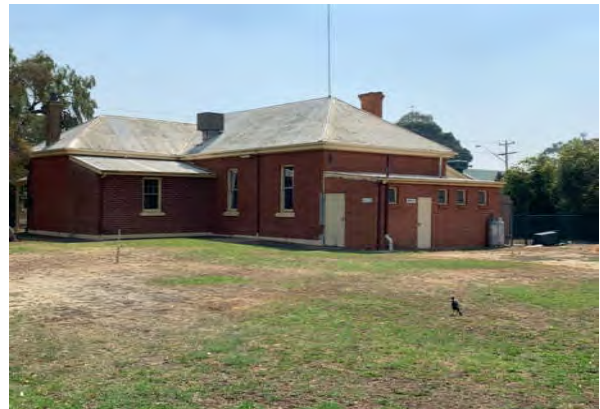
Figure 3D – Rear of existing building
