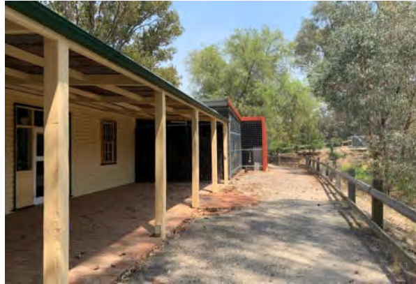
Figure 2B – Existing building (rear)
