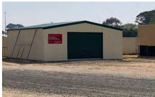
Figure 13 – Machinery storage shed
