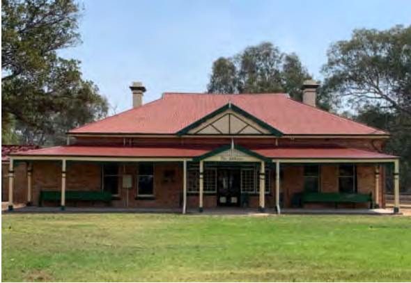
Figure 2A – Existing building (street) 4
