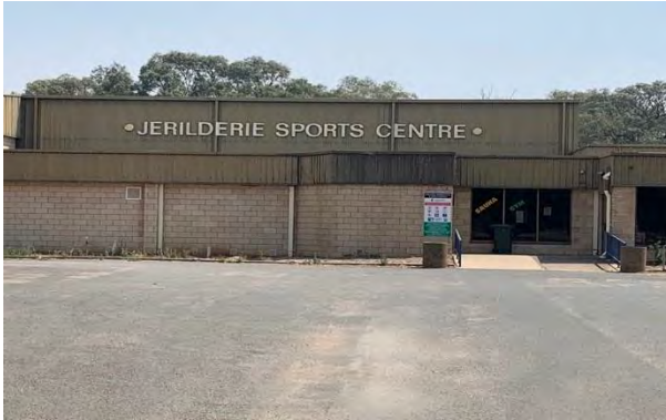
Figure 2 – Main building and carpark 4
