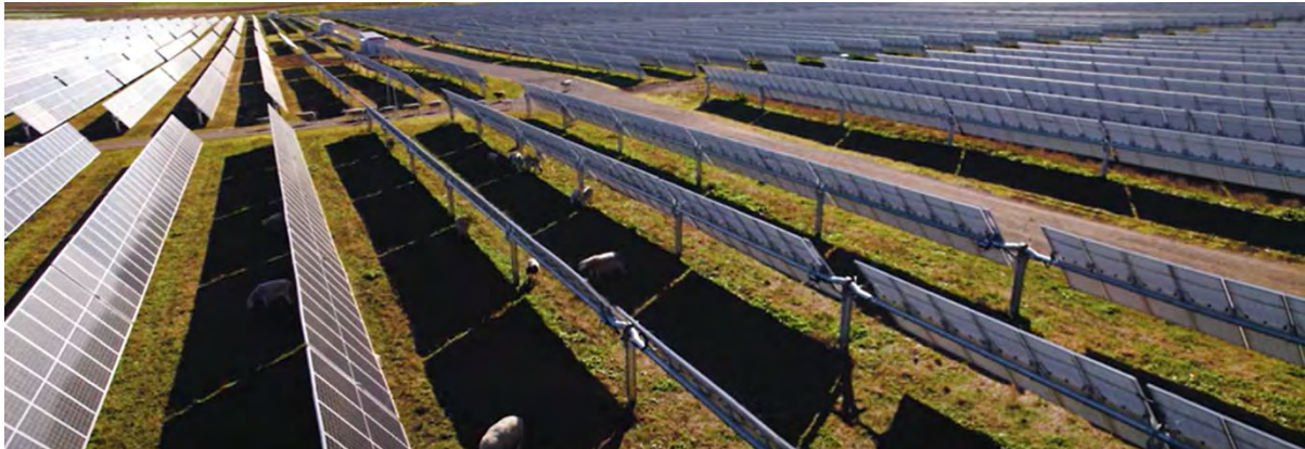
Nextracker SAT system – panels tilted in morning
