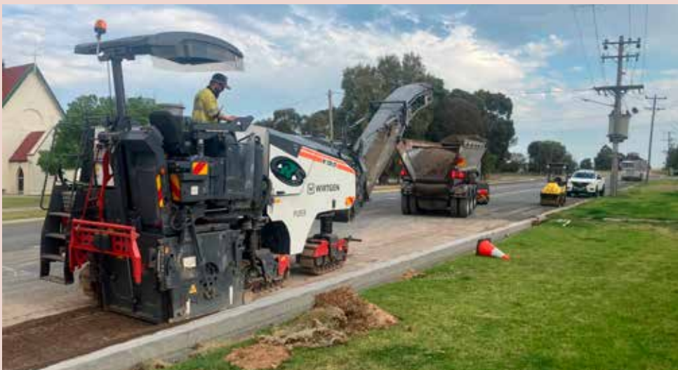
Coreen Street Kerb Removal and Replacement
