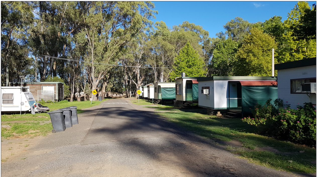
Figure 36: Existing cabin precinct
