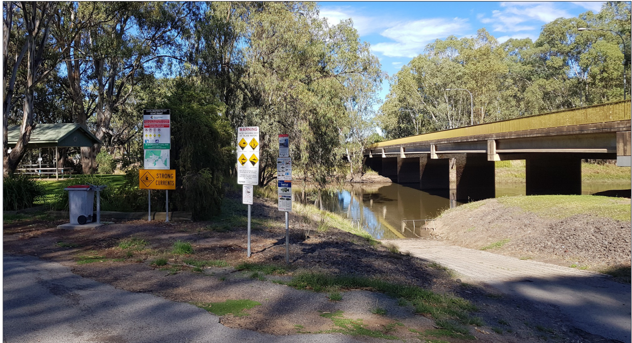
Figure 41: Boat ramp and Lions shelter beside Kidman Way bridge
