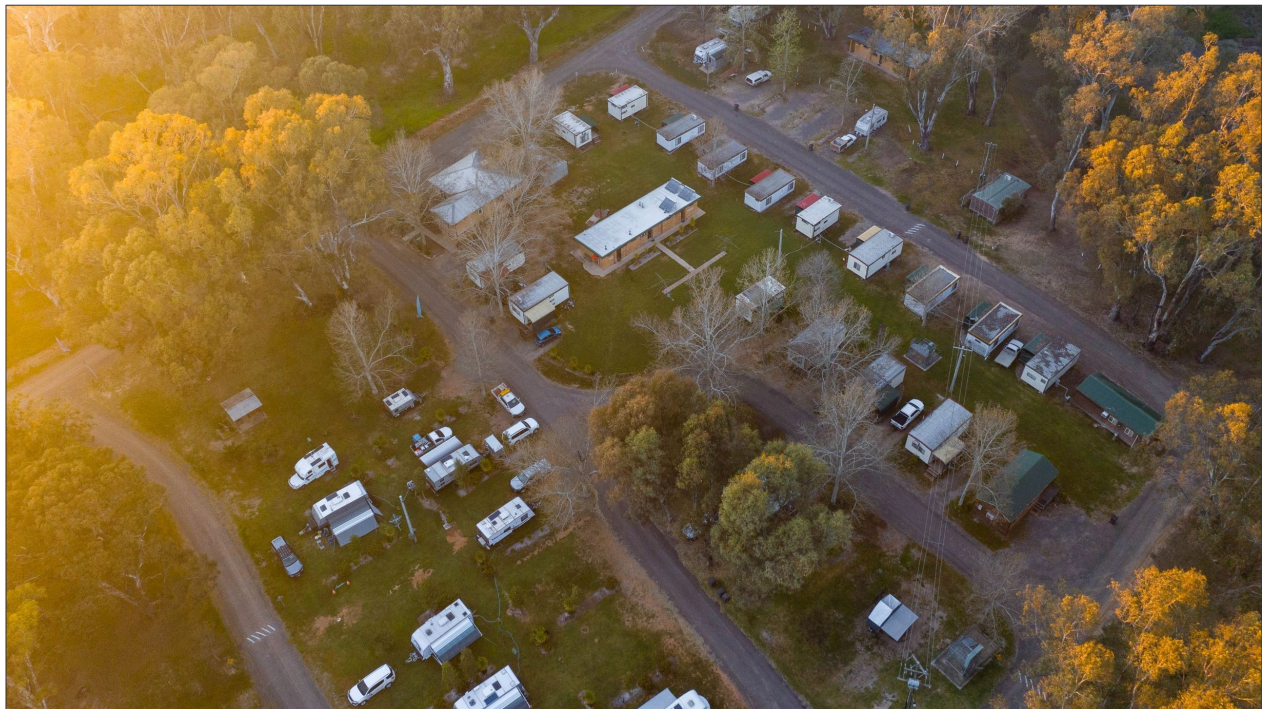
Figure 33: Aerial view of Darlington Point Riverside Caravan Park
