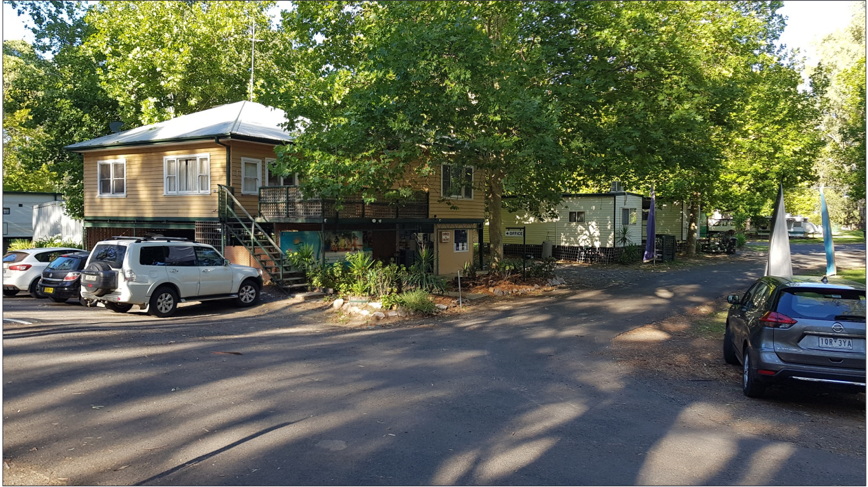
Figure 35: Elevated manager's residence with park office below
