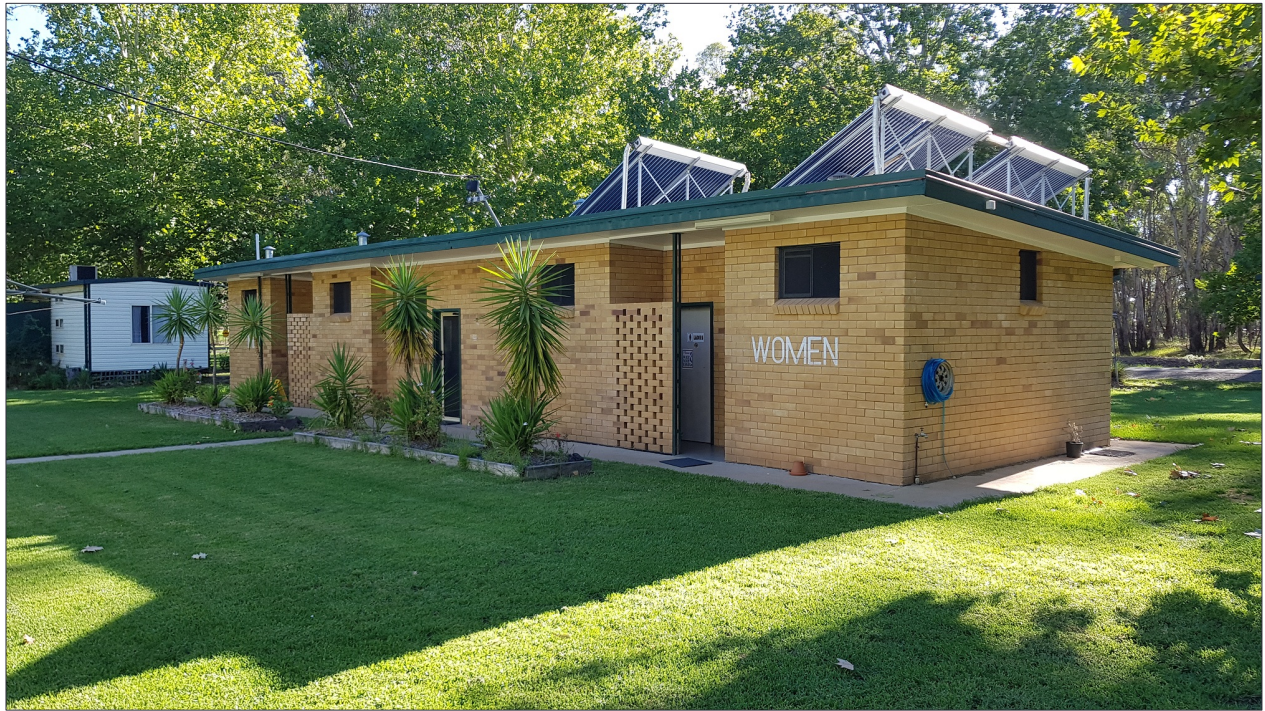
Figure 37: Central amenities building with laundry in the centre
