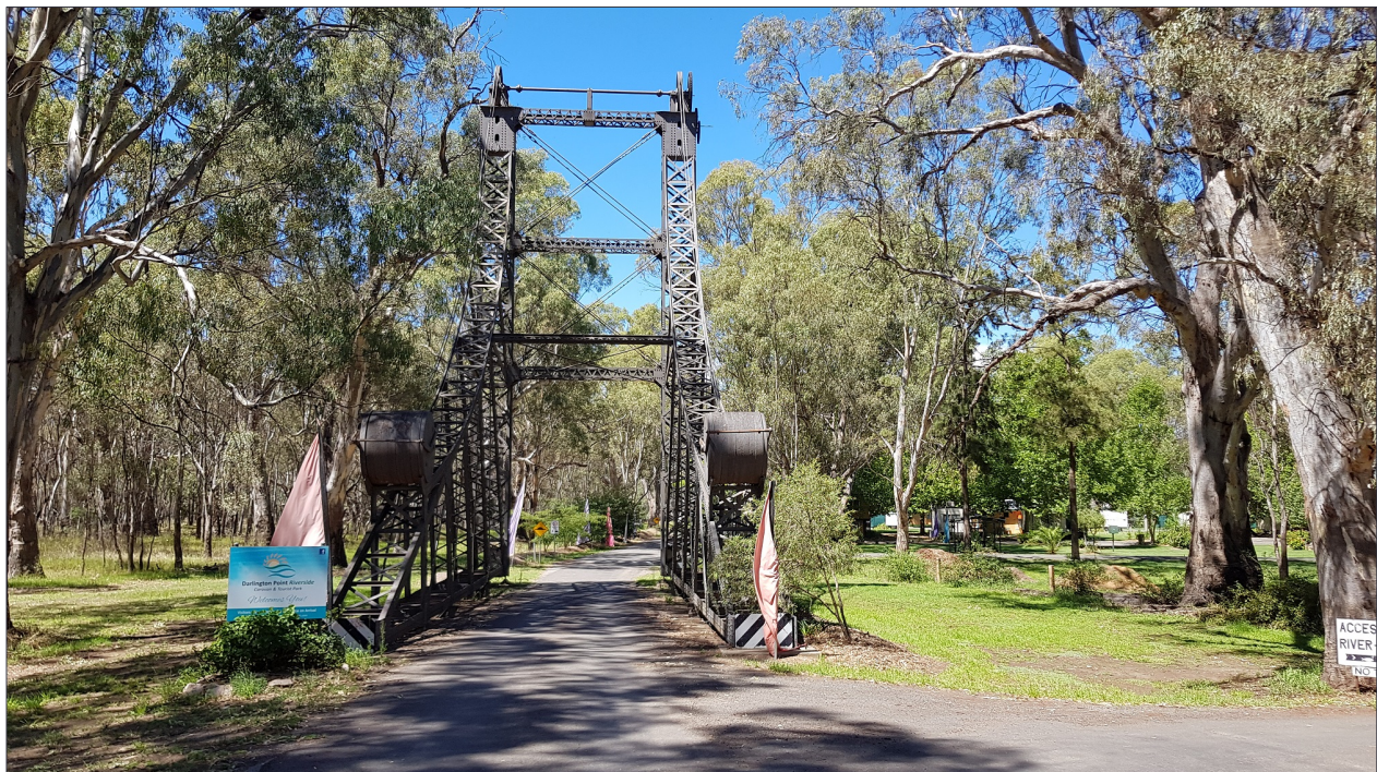
Figure 34: Old Darlington Point bridge at park entry
